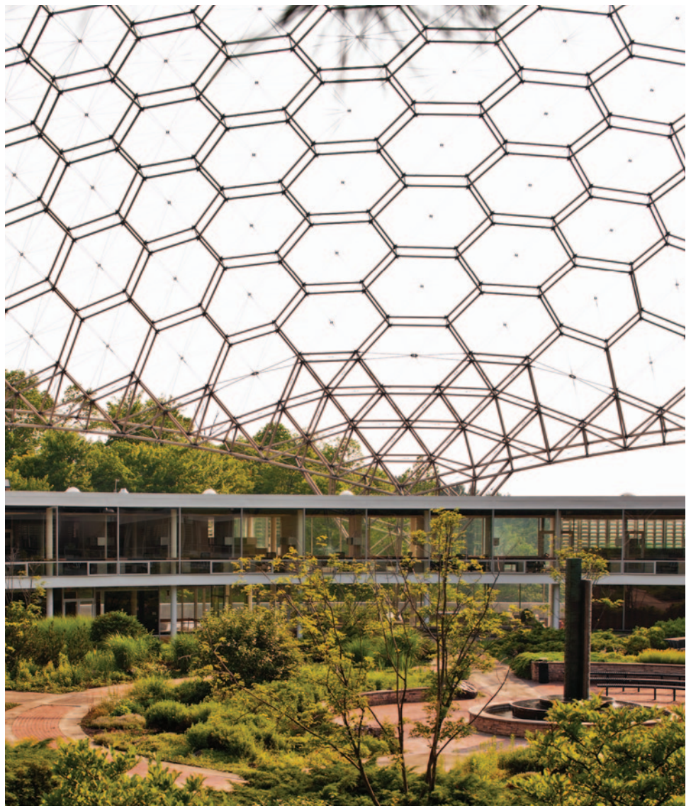
SHAPING THE FUTURE Engineered by R. Buckminster Fuller, the honeycomb-like geodesic dome at ASM International’s World Headquarters is constructed from aluminum alloy tubing and rods in tension, and is supported by five pylons. Still the largest open-work geodesic dome in the world, it stands 103 feet high and 250 feet in diameter, weighing 80 tons.
